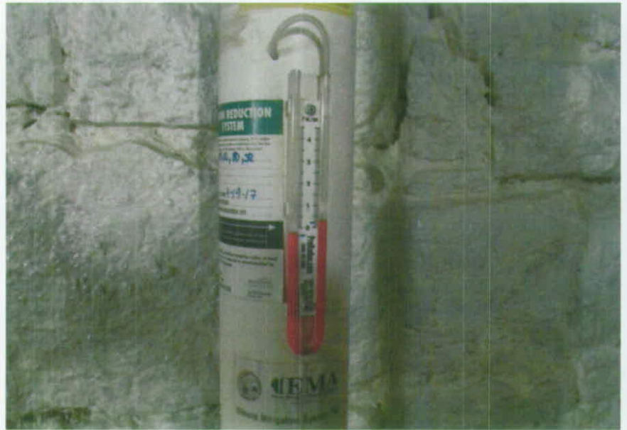
Below: View of SSD Exhaust Piping Extruding from the Basement
